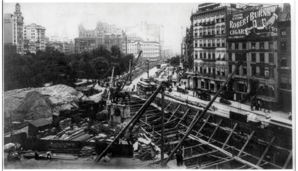
This 1902 photo shows continuing work being done to construct an underground rail system in New York City.
