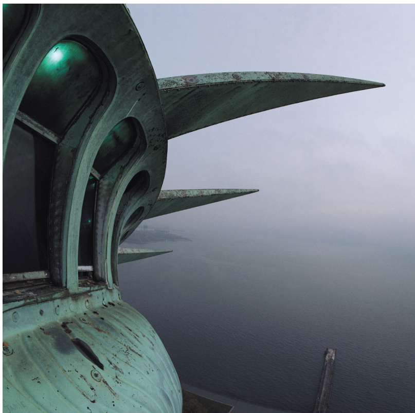
A view from the top of the Statue of Liberty, showing the green patina coating the statue. The patina is formed by corrosion of the copper skin of the statue, which forms a thin layer of an insoluble compound that contains copper(II), sulfate, and hydroxide ions.
