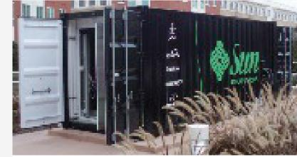
This Sun server-packed container is designed for rapid data center deployment.
