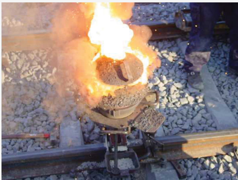
A small clay pot contains a thermite mixture. It is reacting at high temperature in the photo and will eventually produce molten metal to join the railroad tracks below it.
