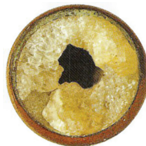
Figure 13.11 Boiler Scale in a Water Pipe
