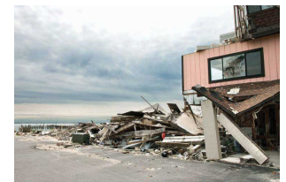
Figure 1.5 A Photo of Galveston Island after Hurricane Ike
