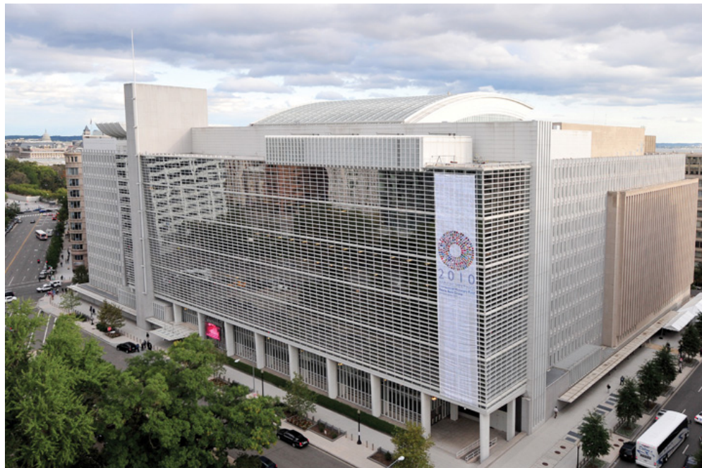
Figure 6.2 World Bank Headquarters in Washington, DC
