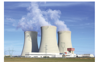
Critics say many US nuclear plants lack adequate protection against several kinds of dangers.
